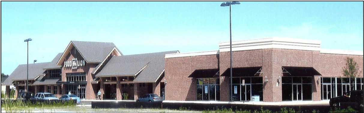
Figure 1. Note the articulation of the larger store to the left and the corresponding lack of articulation on the smaller store on the right.
